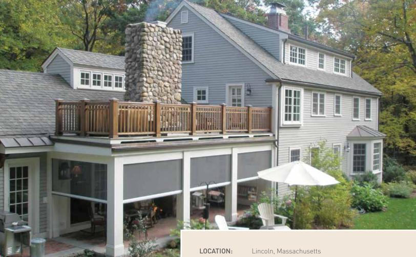
"Phantom's motorized screens retract into cavities designed above the openings, completely hiding them from view. This way the screens don't distract from the simple and elegant design of the porch."
